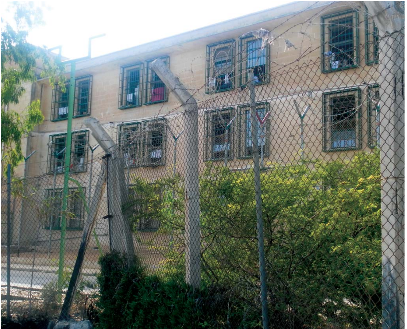
↑ HAL FAR DETENTION CENTRE
